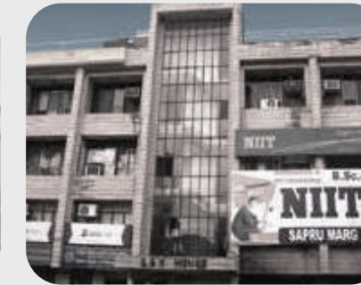
SAS HOUSE SAPRU MARG
