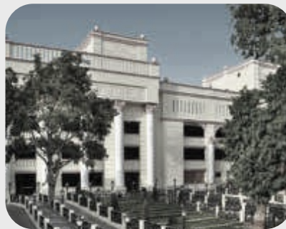
MULTILEVEL PARKING HAZRATGANJ
