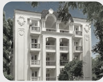
SHALIMAR ROYALE MALL AVENUE
