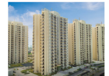
VISTA GOMTI NAGAR EXTENSION LUCKNOW UPRERAPRJ4833
