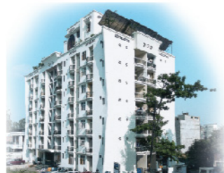
SHALIMAR APARTMENTS P. N ROAD LUCKNOW
