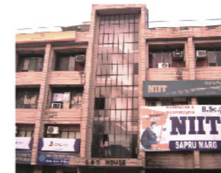
SAS HOUSE SAPRU MARG LUCKNOW
