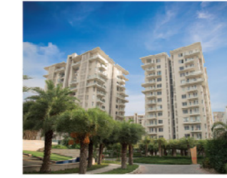
SHALIMAR GALLANT MAHANAGAR LUCKNOW UPRERAPRJ3168
