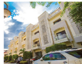
SHALIMAR MEADOWS GOKHALE MARG LUCKNOW
